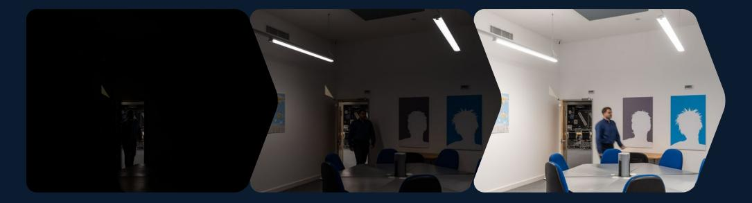
SmartScan Sensors are used to detect movement to turn the luminaires on. After a predetermined time of no movement the luminaires will turn off, saving energy. The sensors can be programmed for absence mode whereby the luminaires are not initially turned on automatically by movement, but manually by the user with a switch; the sensor will then monitor movement to turn the luminaires off automatically after a pre-determined time.
