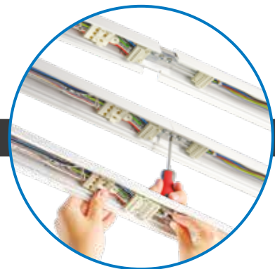
3. Join trunking lengths together
