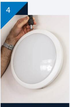
Twist and lock bezel into place and secure with the locking screw.
