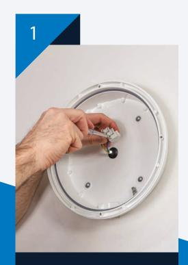
Fix body to mounting surface and install mains connector.
