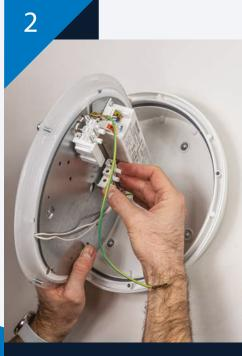
Connect mains connector to mains socket on the LED module.
